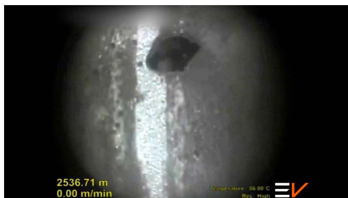
Figure 1: Sideview images of hole in Jet Pump Housing
