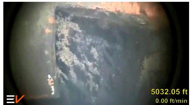
Figure 3: Sideview footage of deformed cut lip guide
