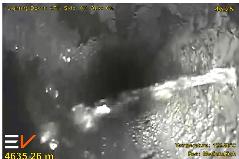
Figure 1: Pin-pointing water entry from a perforation
