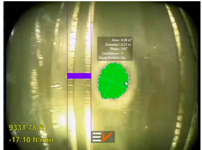
Figure 2: Dimensioned perforation with eroded area calculations
