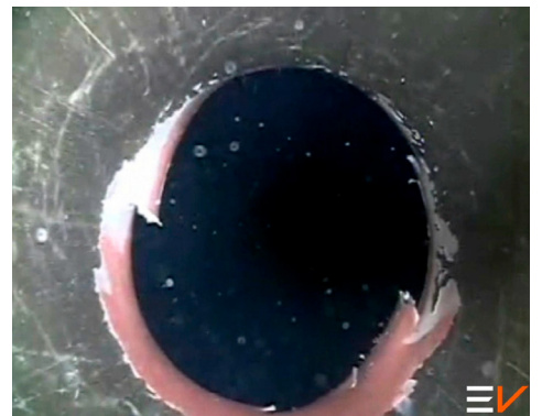
Figure 4: Downview image confirming 11 3/4 inch casing cut
