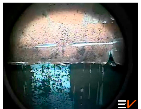
Figure 5: Sideview image confirming final 7 inch casing cut
